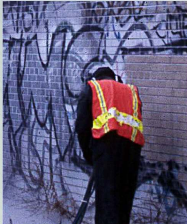
Graffiti removed from brick wall
